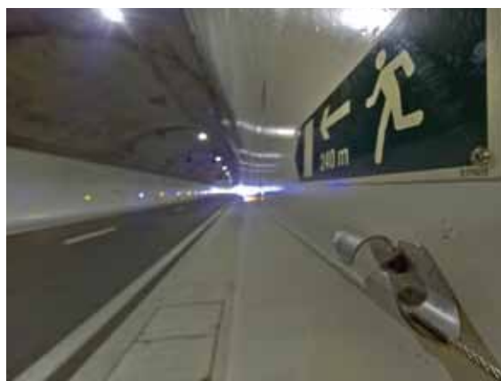
Tunnel de Violay
