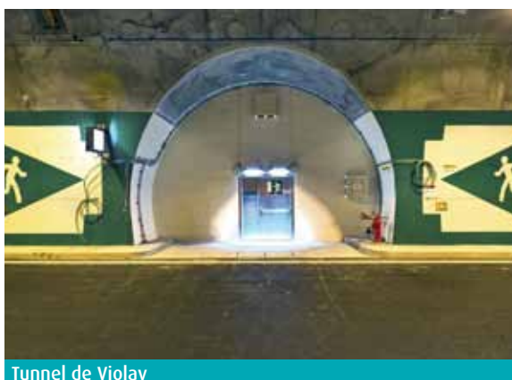
Tunnel de Violay
