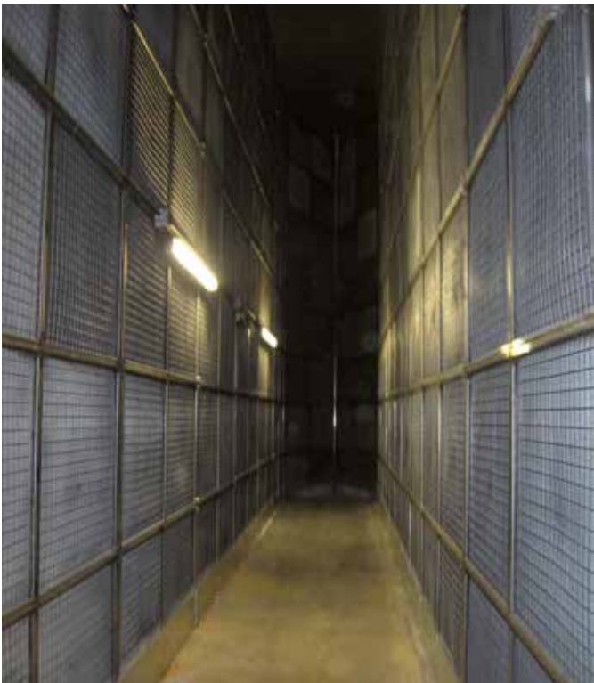
Illustration 30: DeNOx system – air circulates between the panels seen in the photo, a length of several metres is required to ensure a large enough contact surface area
