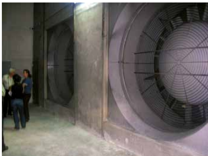
Illustration 17: Extraction fans used for both smoke extraction and air treatment, in horizontal position (cut-and-covered tunnel) – unit characteristics 203 m 3 /s, 630 kW
