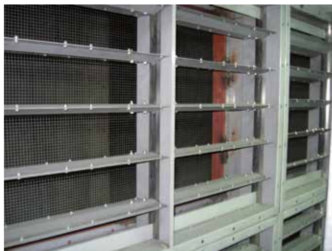
Illustration 20: air treatment circuit intake – close-up of the dampers and pre-filtration meshes (Aigner)
