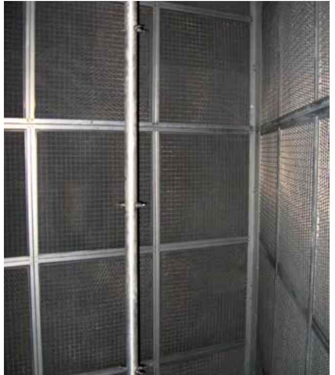
Illustration 27: electrostatic filters and their rinsing nozzles(CTA)
