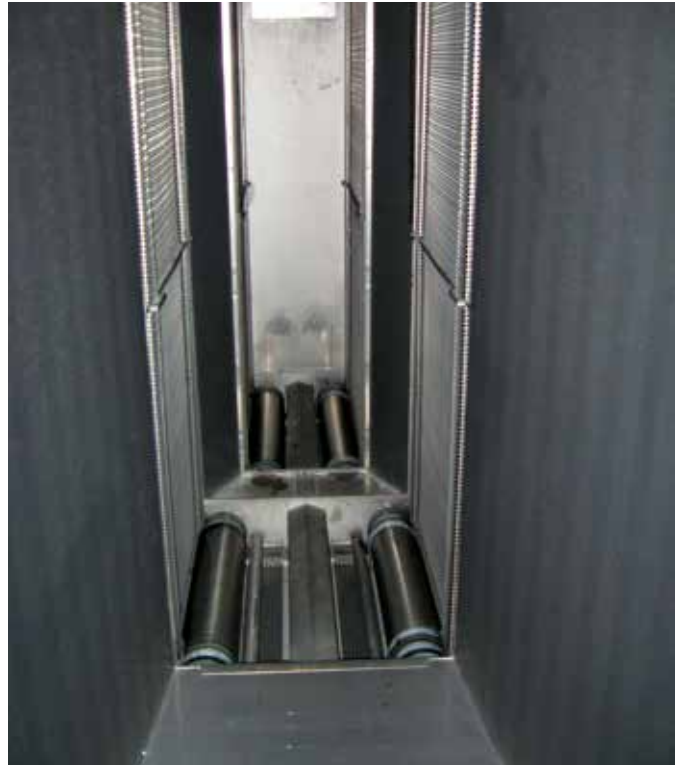
Illustration 24: electrostatic filters mounted on rollers to simplify cleaning under high-pressure air jets (Aigner)
