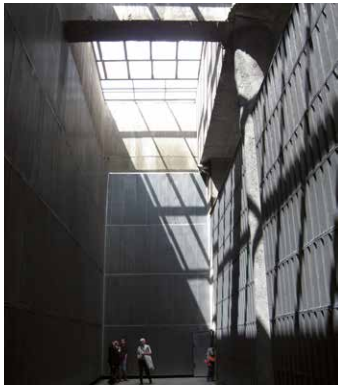
Illustration 32: end of the treatment system (air flows in on the right, fills the plenum then flows out through the opening in the ceiling) – on the right – the acoustic panels demonstrate the size of the aerualics section required to limit flow speeds through the system – at top right, in shadow, the opening that forms the end of the sheathing parallel to the treatment circuit making it possible to short-circuit the treatment system in the event of fire
