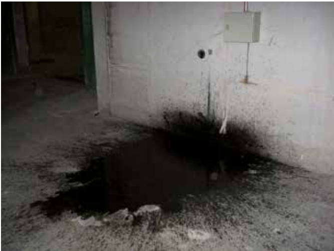
Illustration 39: collection point for treatment residues at the end of the system for treating water used to wash filters (CTA)
