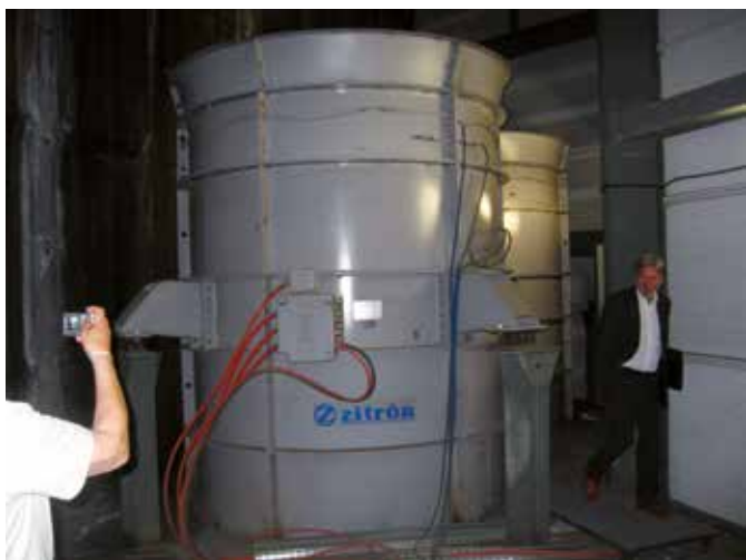
Illustration 18: Extraction fans used for both smoke extraction and air treatment, in vertical position (By-Pass Sur tunnel) – unit characteristics: 116 m 3 /s, 560 kW
