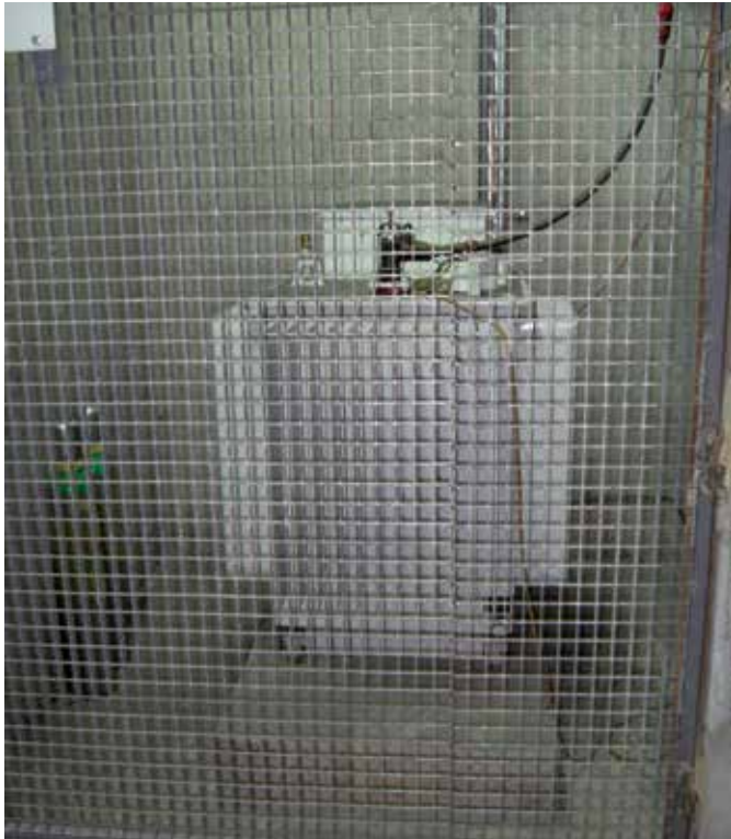
Illustration 33: high-voltage transformer for the ionization current (Aigner)
