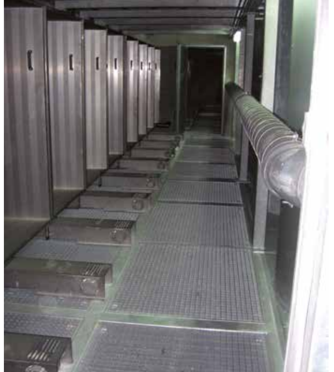
Illustration 23: on the left, cabinets containing the electrostatic filters and, on the right, deNO x system (air circulates from left to right)
