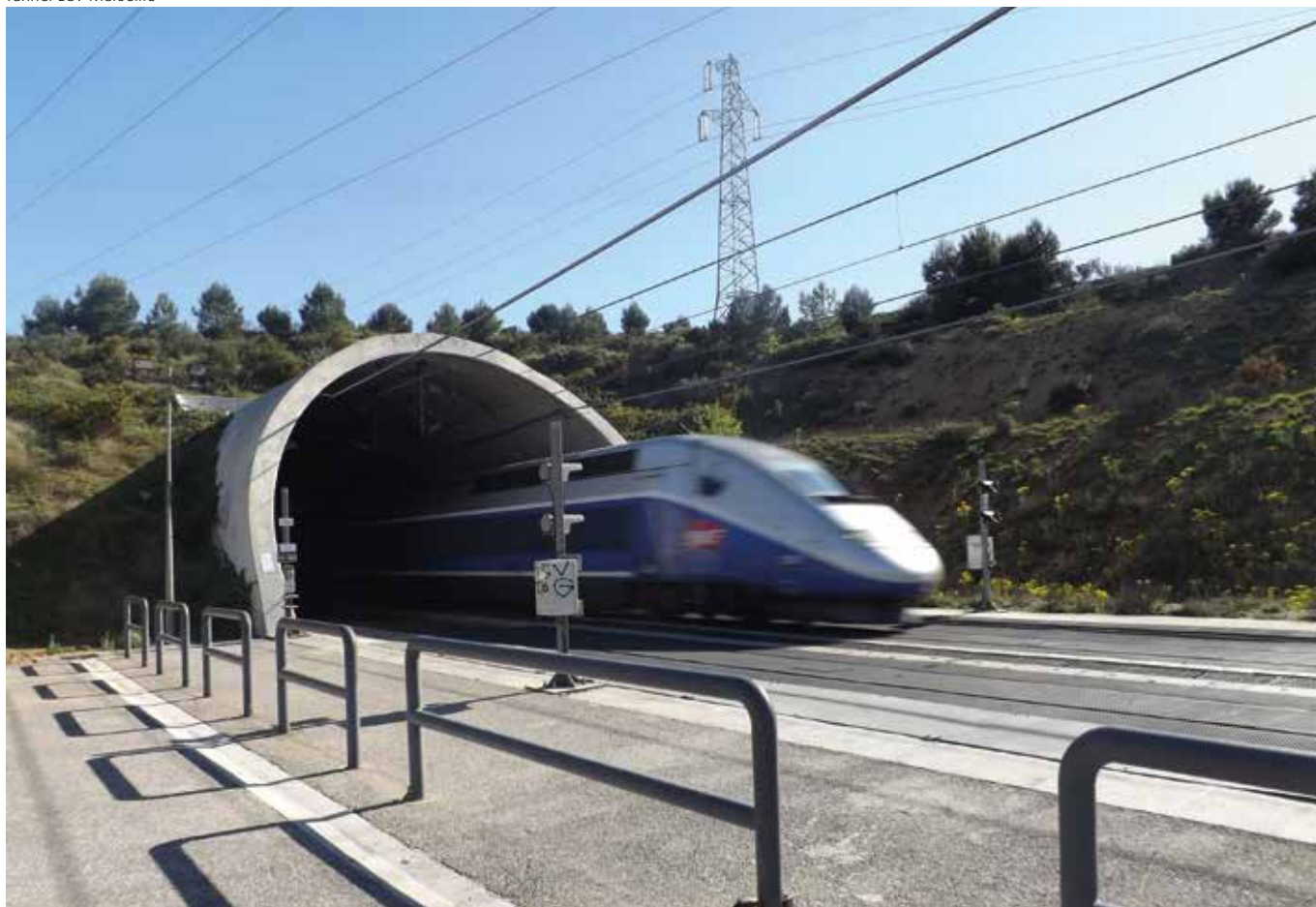
Tunnel LGV Marseille
