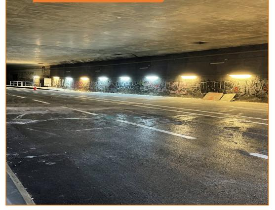
The growing use of LEDs in the tunnel sector and the lack of feedback on their performance in this environment have led the roads directorate of the IIe-de France region (DIRIF) to propose that the unused tube of the Antony cut-andcover tunnel (on the A86 highway) be made available for experimental purposes.
