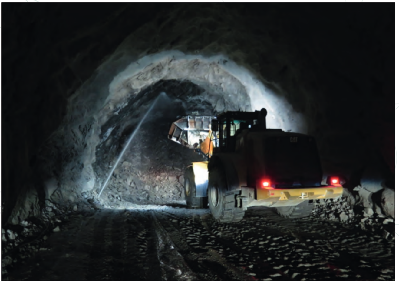
Loading of tunnel muck, Rosten HEPP, Norway. (Photo Ø. Fæhn, Skanska Norge AS)
