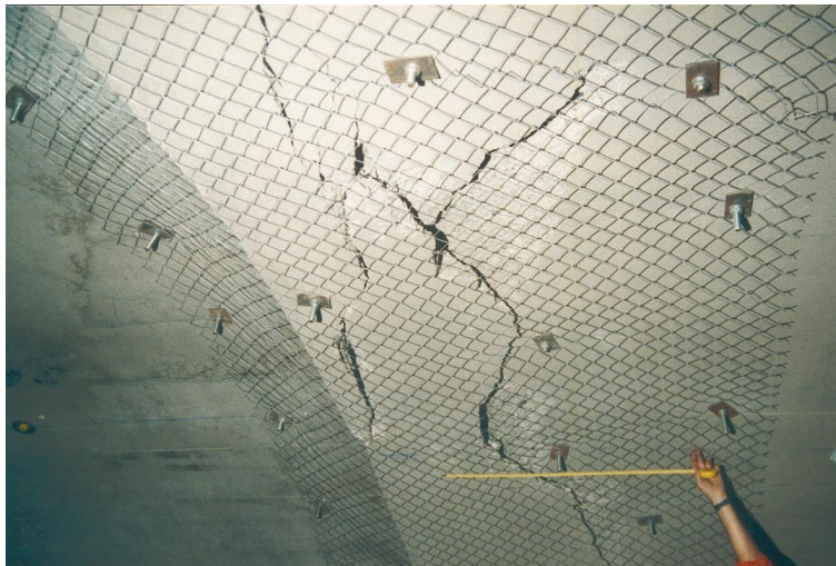
Figure 3: rupture of a reinforced cast concrete arch under the action of stresses that are too high
