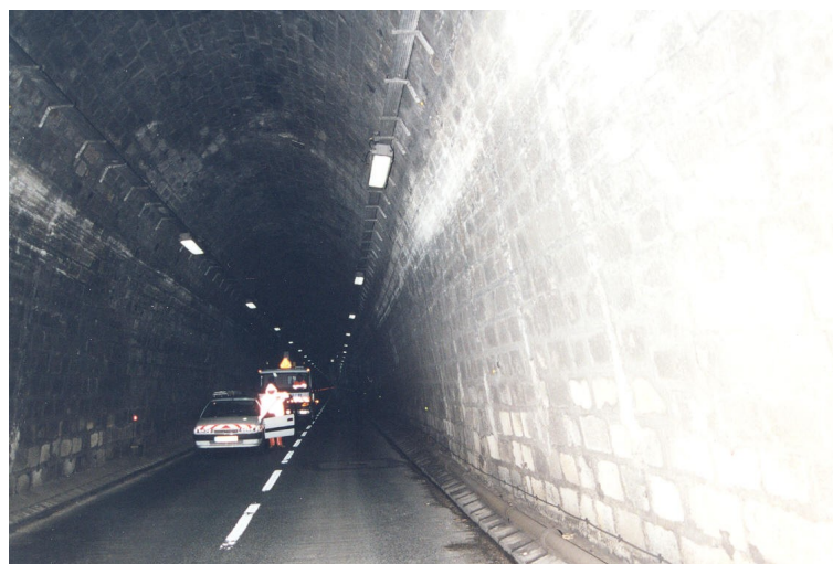
Figure 5: asymmetrical squeezing (the light part has lost its original curve)
