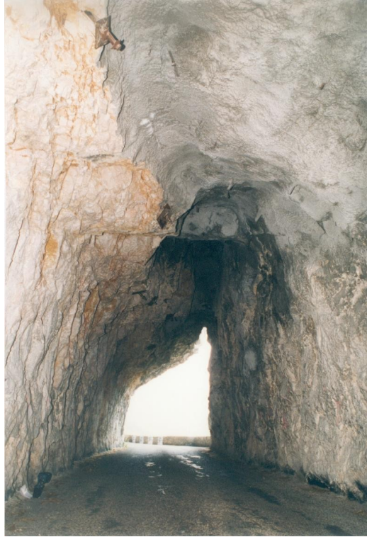
Figure 3: residual instabilities reinforced with sprayed concrete in the lateral reaming area
