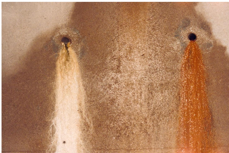
Figure 3: light calcite concretions (on the left); red gel deposit, rich in iron oxide (on the right)
