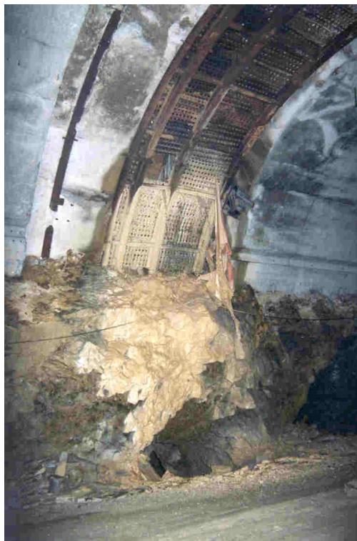
Figure 1: limestone concretions encrusting the opening of an active karst in an abandoned tunnel
