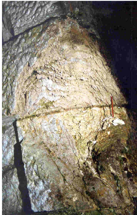
Figure 1: effects of freezing on large oolitic limestone stones
