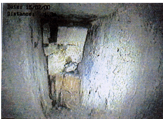
Figure 2: examples of drainage channels blocked with site debris (video-endoscopy)
