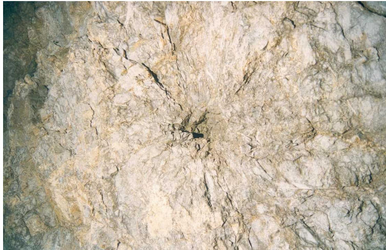
Figure 1: limestone excavated at the beginning of the 19 th century [fractures can be seen radiating from a blast hole; the entire rock is loosened and unstable]
