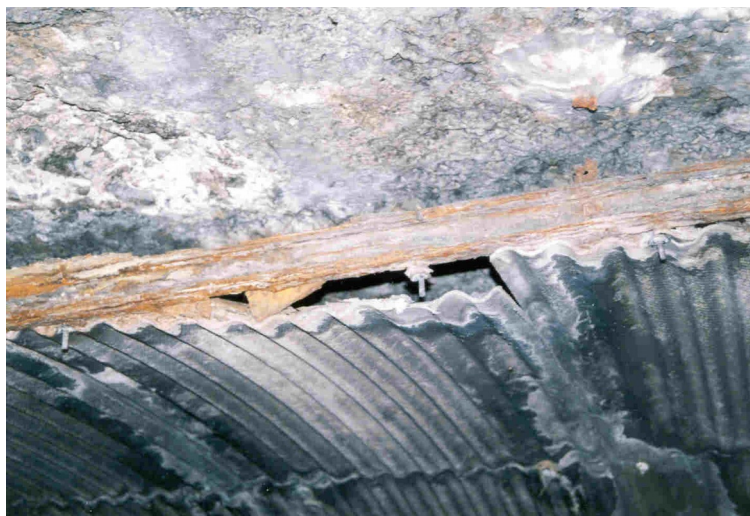
Figure 2: fibre-cement panels (significant oxidation of the support rails and an element which has become unfixed)
