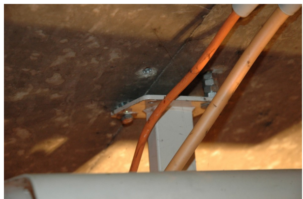
Figures 2a and 2b: partially or totally severed cable tray hangers or camera fastenings
