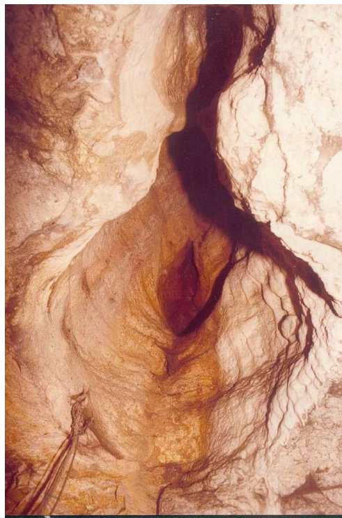
Figure 2: open conduit leading to the roof section of an unlined tunnel (traces of temporary flows mixed with red clay can be seen)
