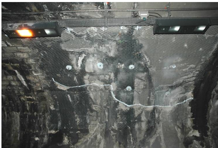
Figure 3: rupture of a reinforced cast concrete arch under the action of stresses that are too high
