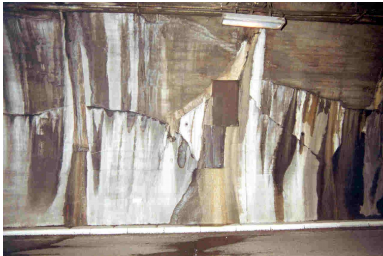
Figure 2: development of shrinkage in concrete from 1970 without a waterproof membrane applied to the extrados
