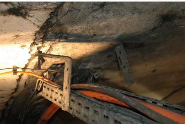
Figures 2a and 2b: partially or totally severed cable tray hangers or camera fastenings
