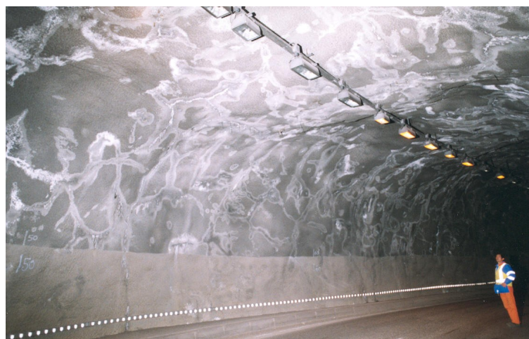
Figure 2: same tunnel after a few years in operation
