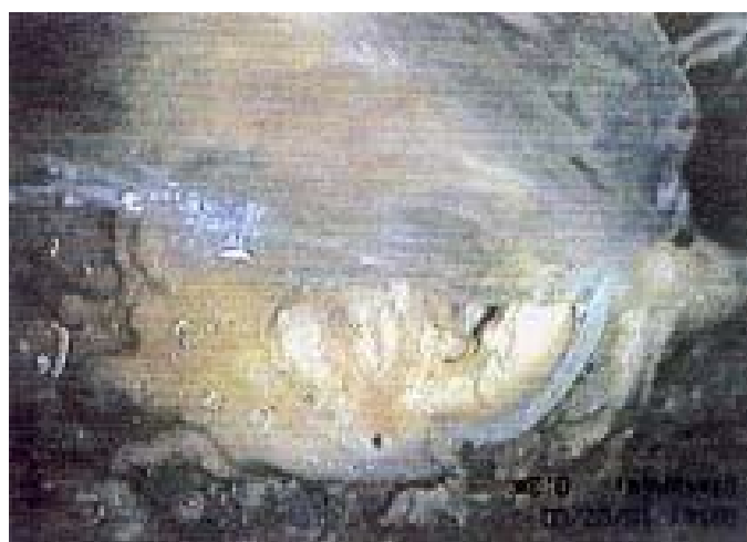
Figure 2: video-endoscopy of a PVC drain blocked with calcite
