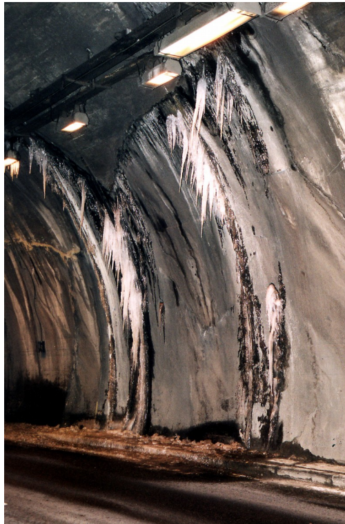
Figure 2: stalactites and packs of ice on the ground
