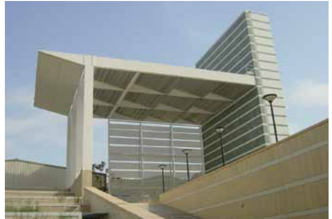
Photo 5 - the UV2 ventilation unit in the Toulon tunnel
