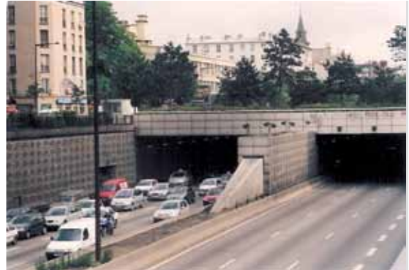
Photo 7 - Central dividing wall – Landy cut-and-cover tunnel – A1 motorway (Seine Saint Denis)
