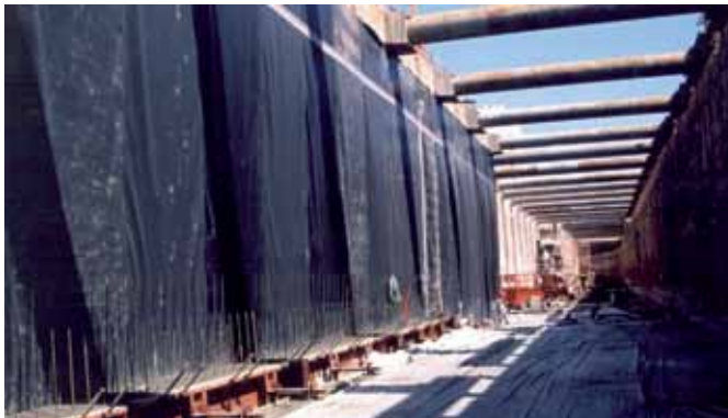
Photo 3 - Cut-and-cover tunnel under construction (Toulon Underpass)
