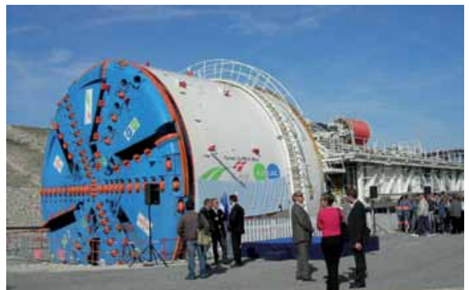
Photo 2 - Rotary digger shield excavating the Mont Sion tunnel (A41)
