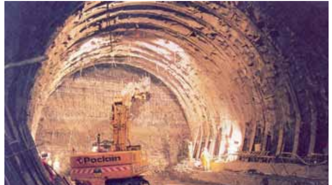
Photo 1 - Excavation by traditional method
