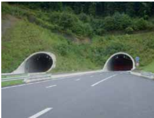
Photo 6 - Offset portals – Uriol tunnel on the A51 motorway
