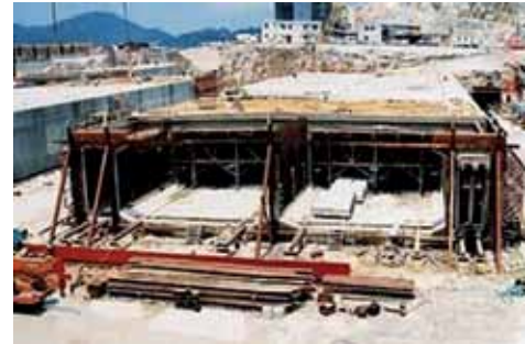
Photo 4 - Tubes under construction
