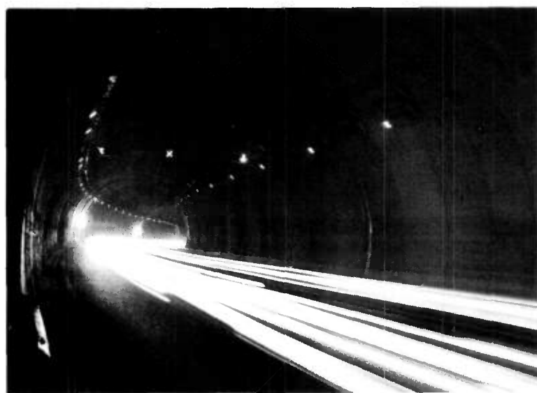
Figure 38. Autoroute A. 8. - Tunnel de la Baume.
