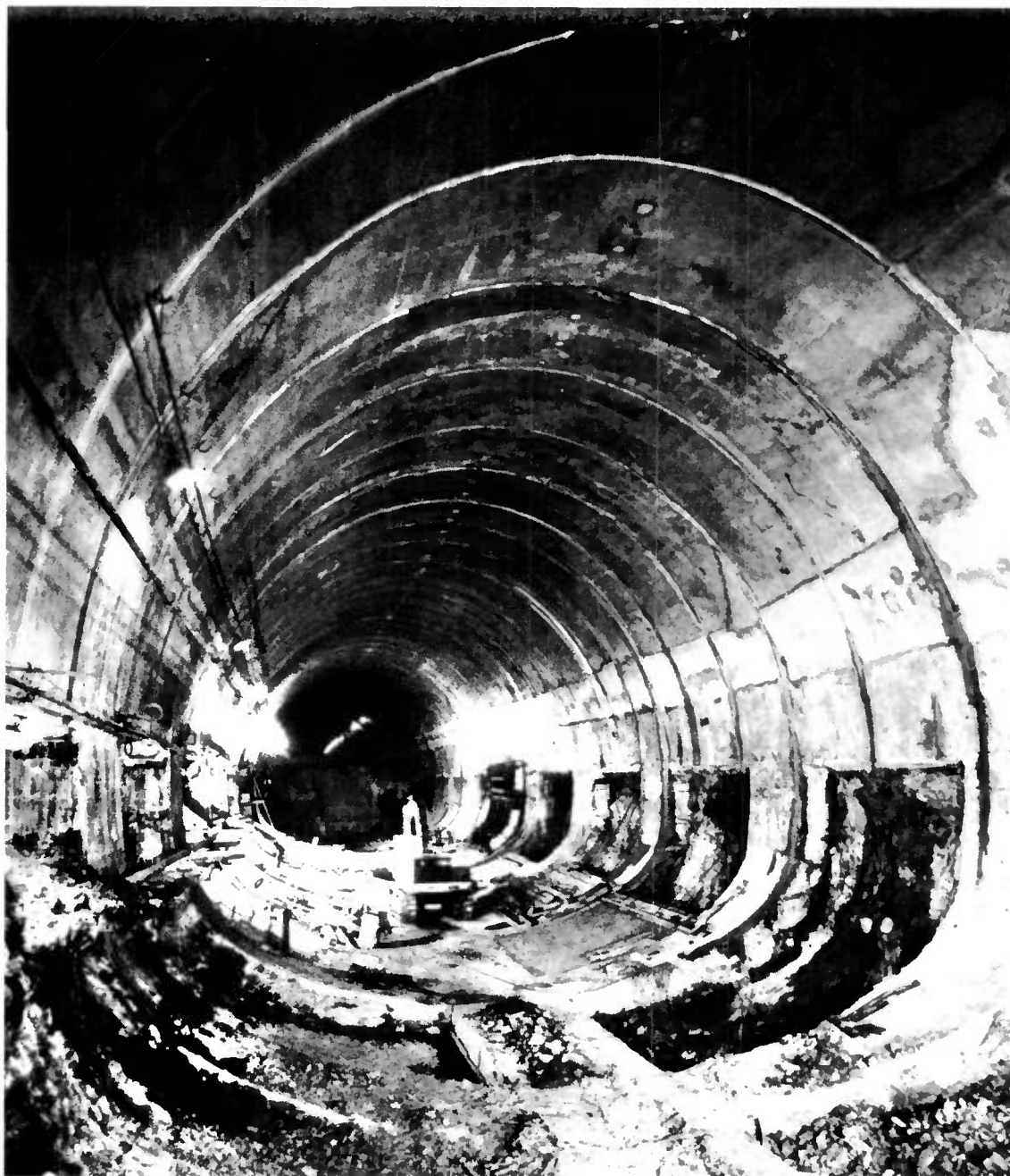
Figure 12. Tunnel André Malraux (Cimiez) - Nice.
