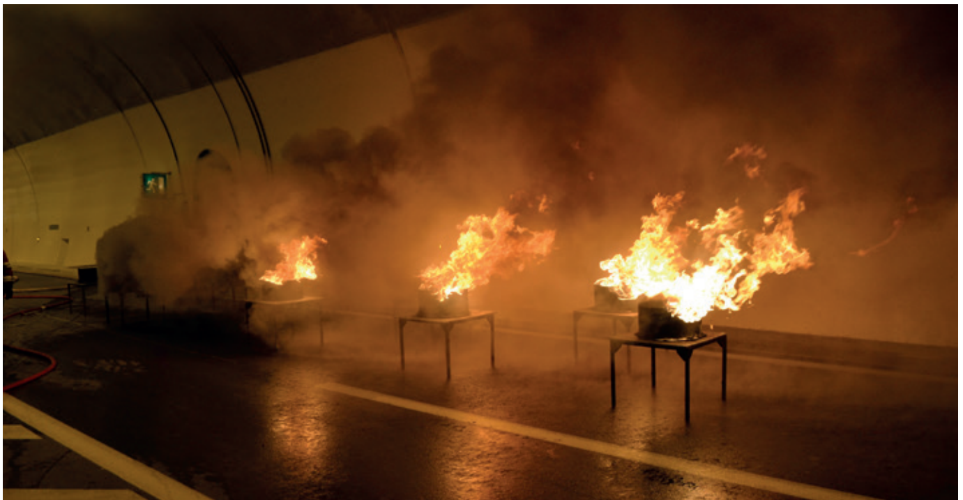
Talant Tunnel – Fire test (© CETU)
