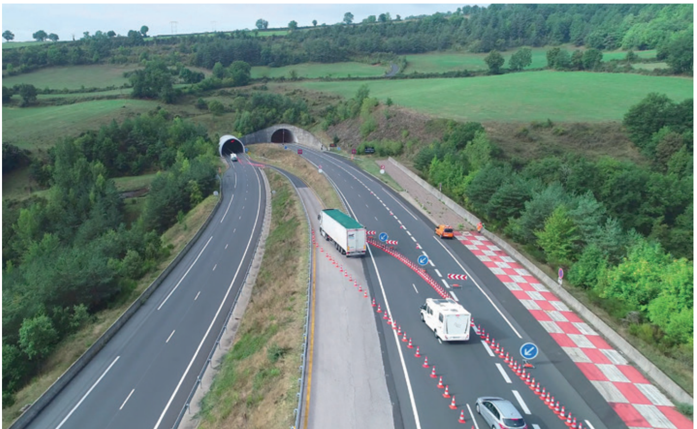
Entrance to the Montjézieu tunnel (© DIRMC)
