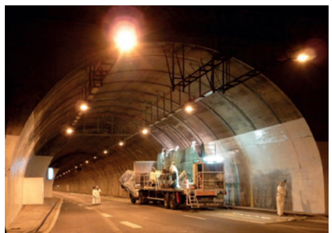
Rond-Point Tunnel – Painting works (© CETU)
