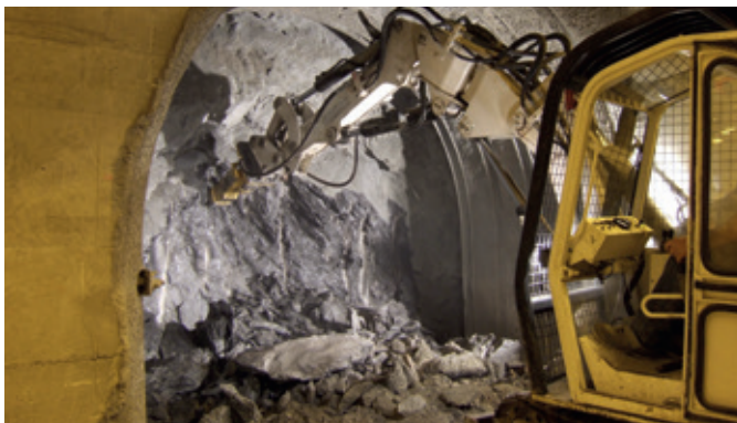
Rond-Point Tunnel – Intertube drilling work (© CETU)
