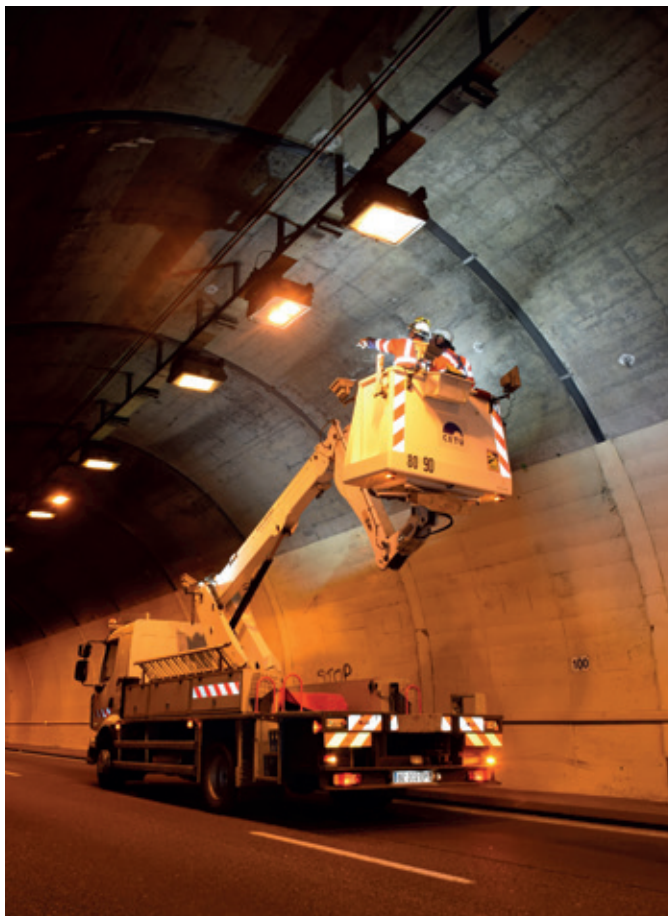
Rond-Point Tunnel – Periodic detailed inspection of structural elements (© CETU)
