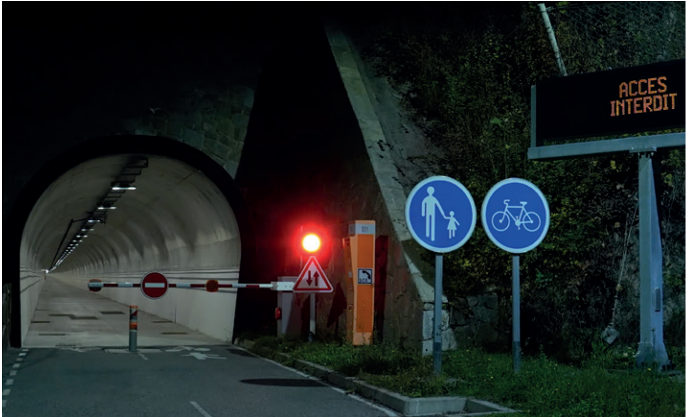
Siaix Tunnel – Safety exercise 2024 (© DIRCE)
