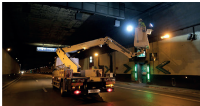
A14/A86 complex – Detailed periodic inspection of equipment (© CETU)
