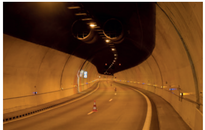
Ponserand Tunnel during a periodic detailed inspection of structural elements (© CETU)
