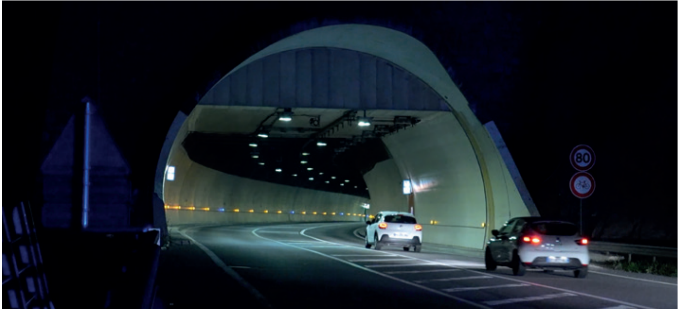
Siaix Tunnel – Safety exercise 2024 (© DIRCE)
