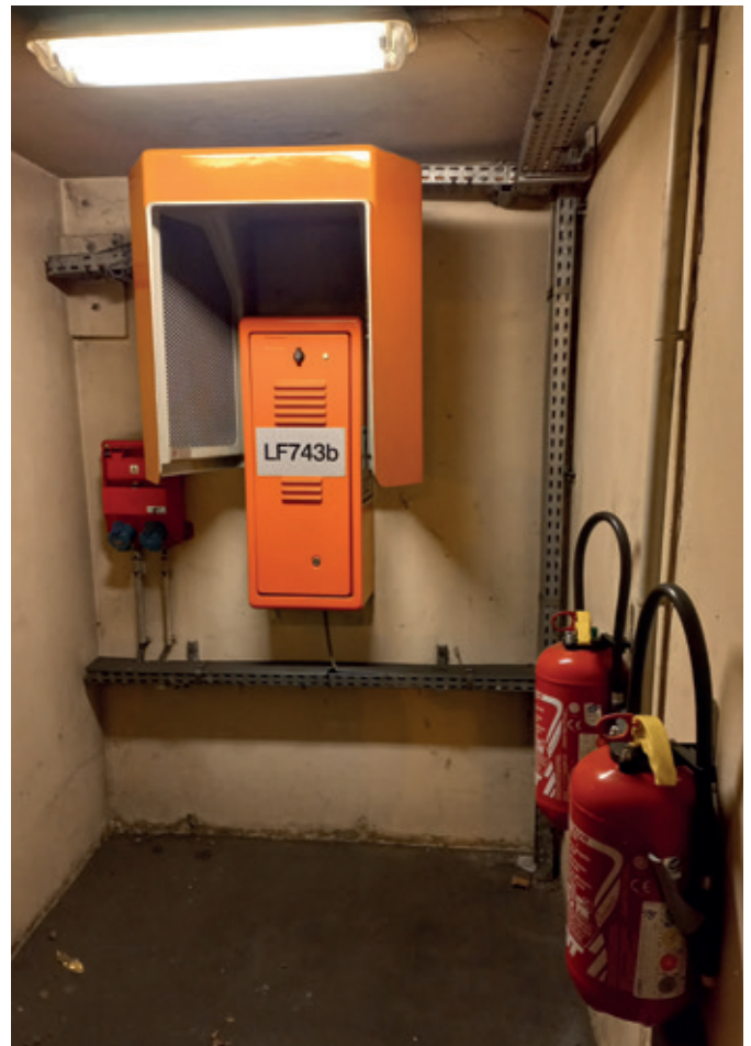
Lilas cut and cover tunnel – Emergency exit (© City of Paris)
