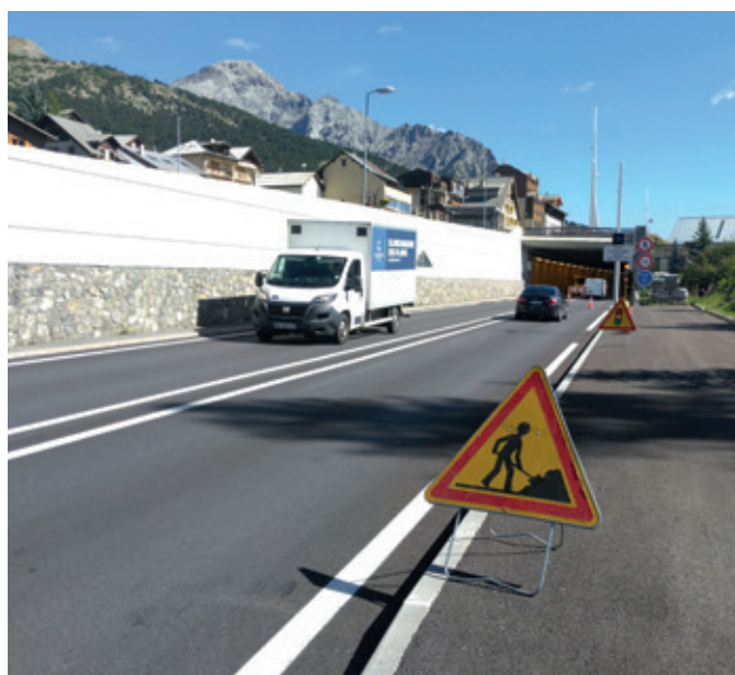
Montgenèvre cut and cover tunnel (© DIRMED)
