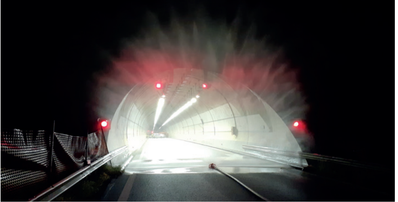
Entrance to the Noailles tunnel (© DIRCO)
