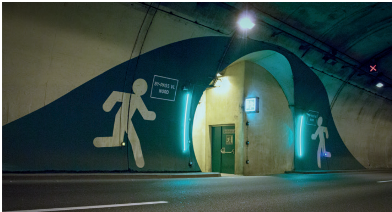
Grand'Mare Tunnel – Explanatory emergency exit (© CETU)
