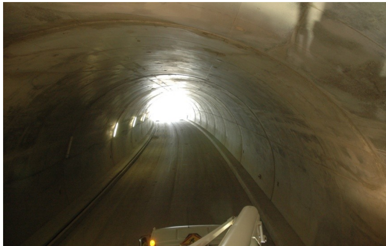
Figure 8: un-reinforced concrete lining
