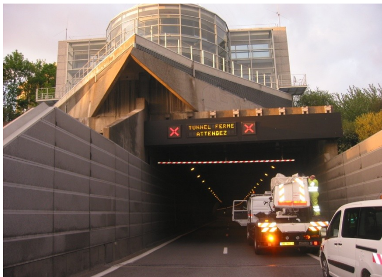
Figure 5: ventilation plant at the tunnel portal
