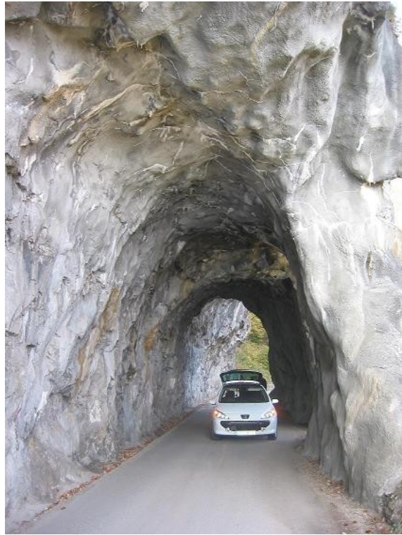
Figure 7: Unlined tunnel
