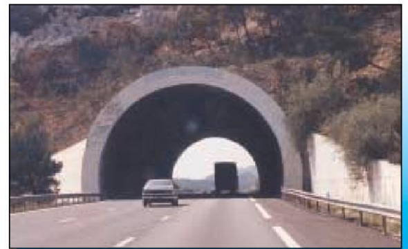
Langesse Tunnel on the A8 motorway (the “visible exit” criteria is respected)
