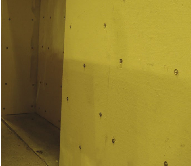
Board type fire protection
