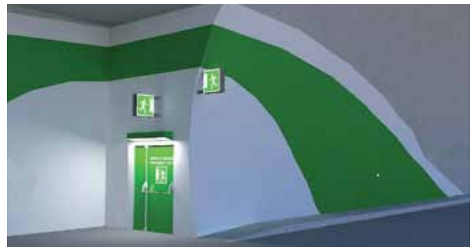
Figure 5: Example of layout of emergency exits located at the back of garage.
