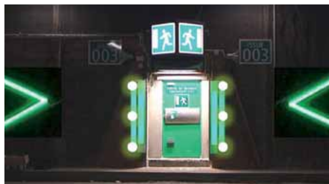
Photo of the mock-up
