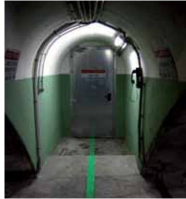
The green line on the floor effectively guides the user outside the tunnel. The bottom of the wall painted in green reinforces the efficiency of this guidance.
