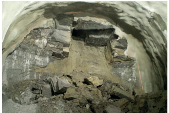
Figure 4: Example of instability in rock mass in the Chavannes tunnel (France).
