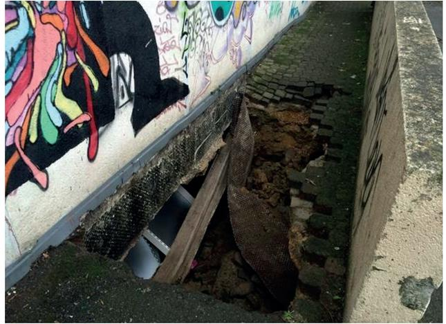
*Photograph of the sinkhole that appeared in the Noz store. It has a surface area of about 20 m<sup>2</sup> and is 3 m deep. Three people fell into this sinkhole, but were able to get out of it without serious injury.*
