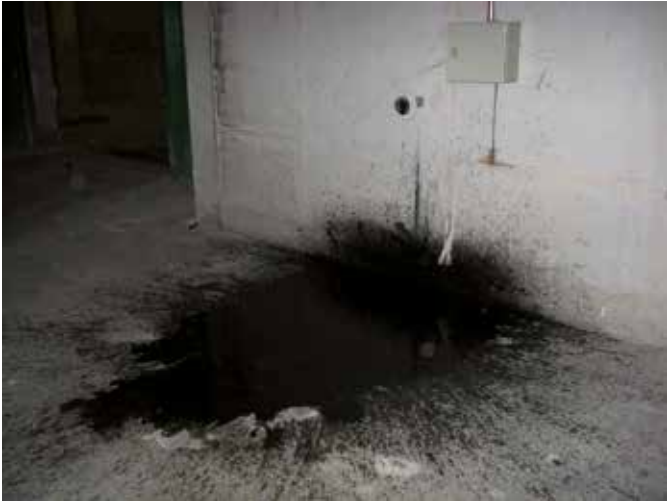
Illustration 39: collection point for treatment residues at the end of the system for treating water used to wash filters (CTA)
