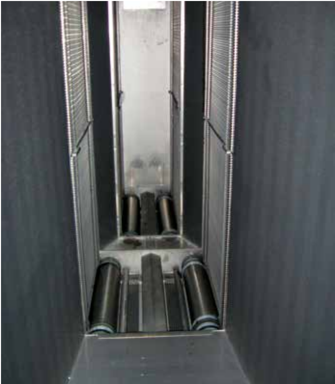
Illustration 24: electrostatic filters mounted on rollers to simplify cleaning under high-pressure air jets (Aigner)
