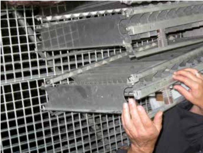
Illustration 22: components of the ionisation system
