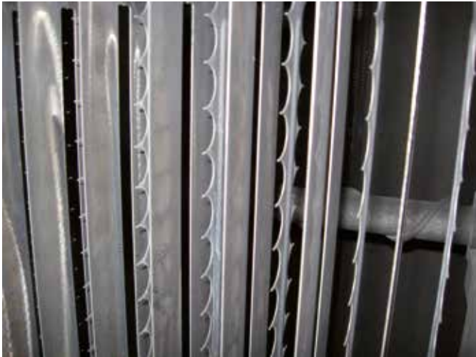
Illustration 21: ionisation device – the difference in potential is established between the points seen in the photo, air is electrically charged on passing between the blades
