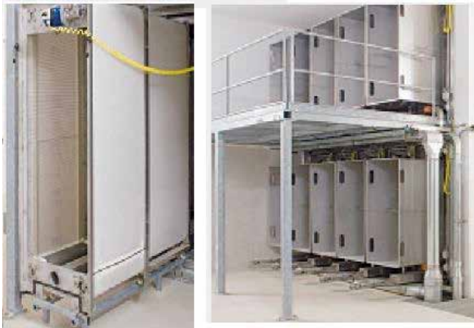
Illustration 8: example of basic filtration modules alone (left) and in series (right) (Source: http://www.aigner.at )
