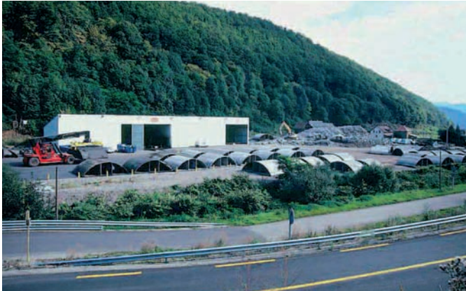
Photo 15: treatment unit (source: Thiboud A, Tournery H. et Duteil A, Travaux n°855 – September 2008, [34])
