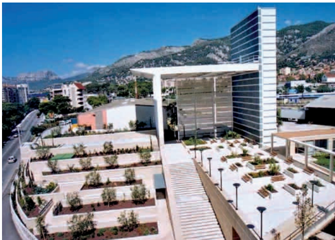
Photo 11: ventilation unit UV2 in the Toulon tunnel (source : CETU)
