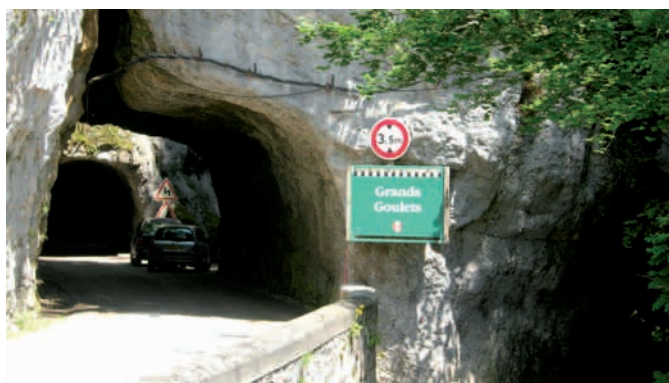
Photo 23: former Grands Goulets road in the Vercors (source: CETU)
