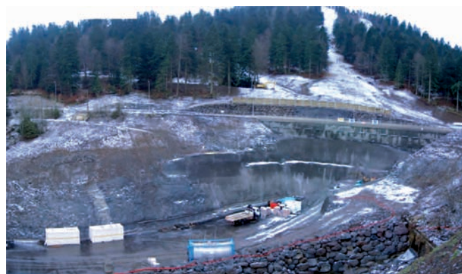
Photo 9: worksite at the North portal of the Lioran tunnel (source: CETU)
