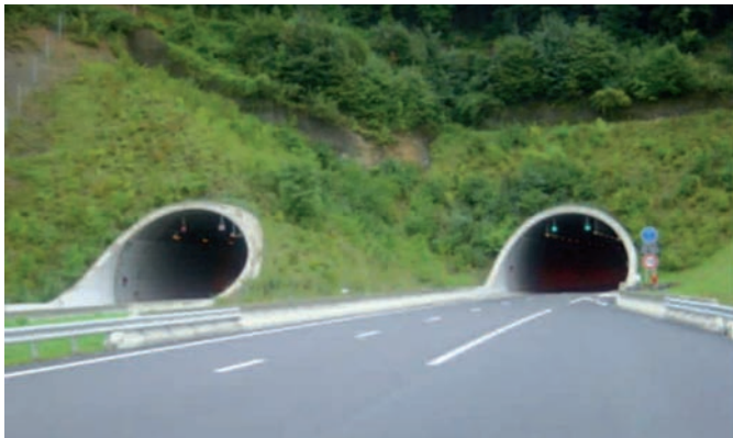
Photo 8: Uriol tunnel on the A51 motorway (source: CETU)
