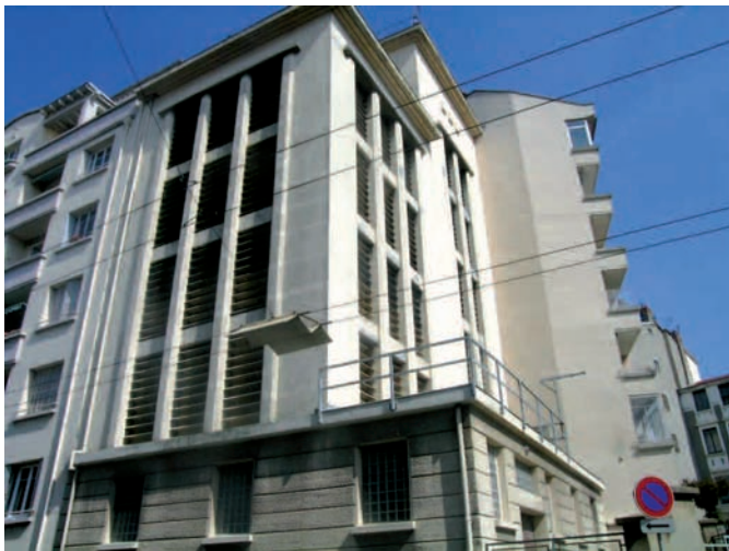
Photo 4: stack at the Croix Rousse tunnel opening onto Croix Rousse plateau (source: CETE de Lyon)
