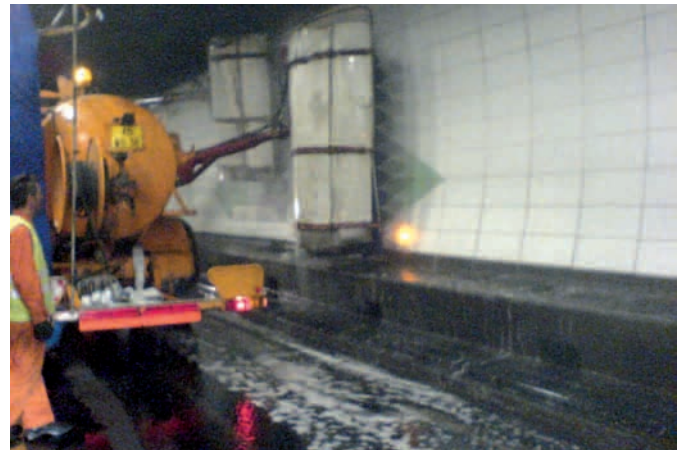
Photo 17: rinsing operation in the Fourvière tunnel in Lyon (source: CETU)
