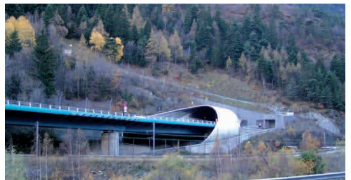
Photo 5: tunnel portal extended by a tube – A43 motorway in Maurienne (Orelle) – Apart from its landscaping advantage, this type of solution can be used to offset the emission source by a few tens of metres (source: CETE Lyon)
