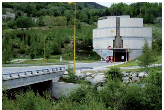
Photo 25: Puymorens tunnel in the Pyrenees (source: CETU)
